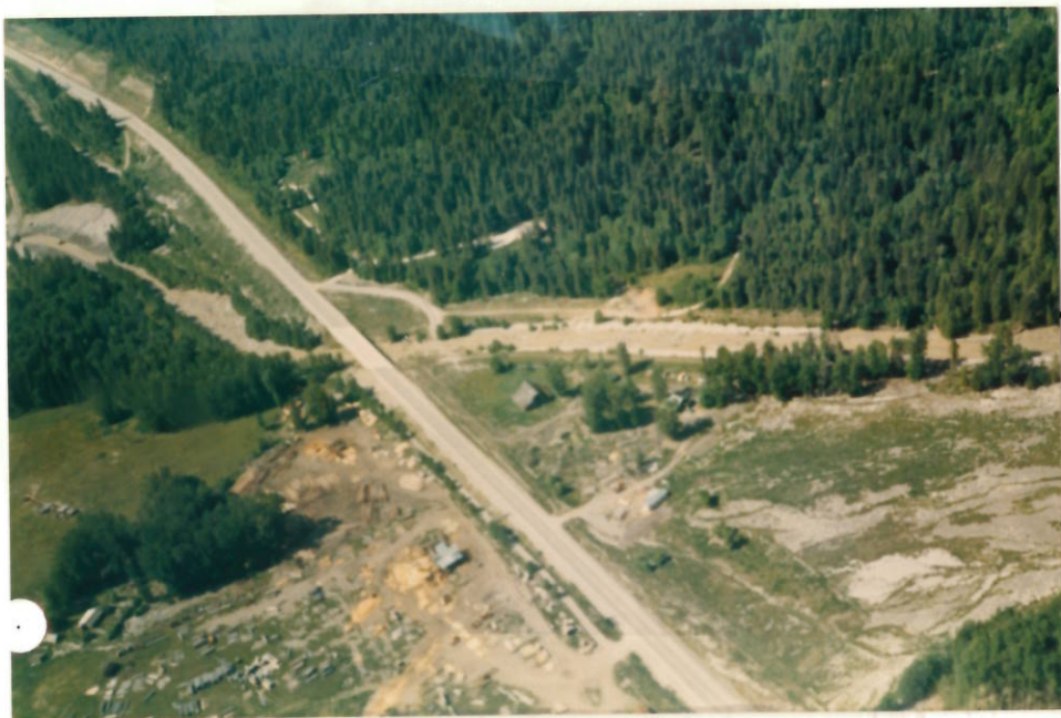
Photo #2 - Flow moving around house.
